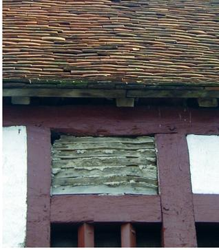
Cleft oak or chestnut 'laths' were sometimes nailed across the staves, as for North Cray, though, this construction is considered less usual. Lath eventually became common when plaster superseded daub from the 18<sup>th</sup> century.
