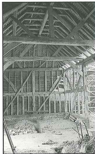
The interior of Cowfold Barn before it was dismantled.
