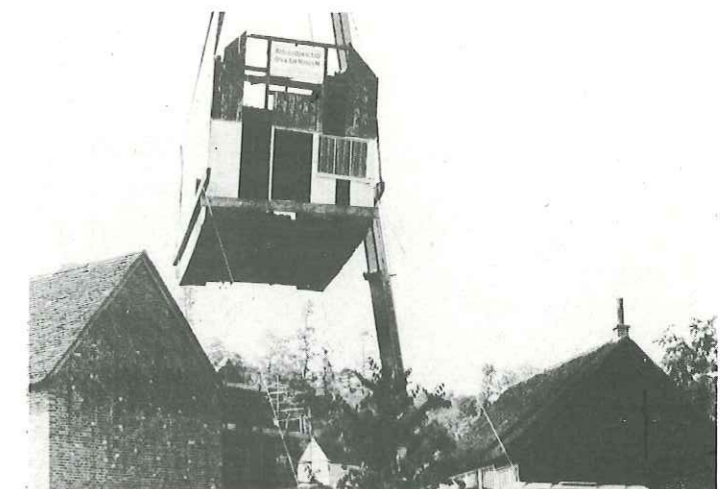
The building is hoisted into position behind the Museum Shop.
