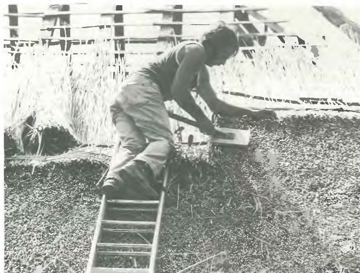
PHOTO- Thatching of Court Barn Rod Miller of South-western Thatchers
